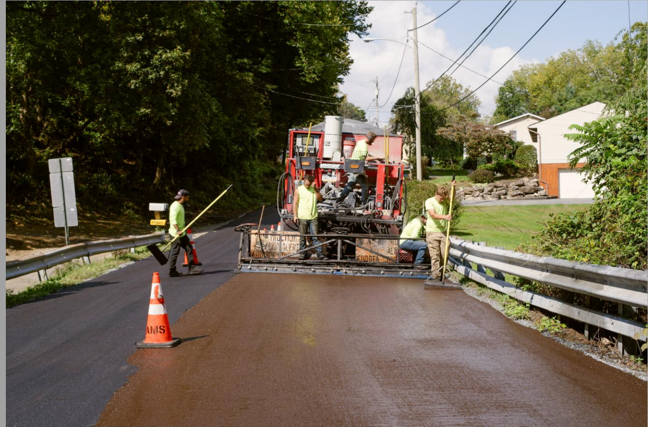
Quick Set Type II Slurry over Chip Seal
