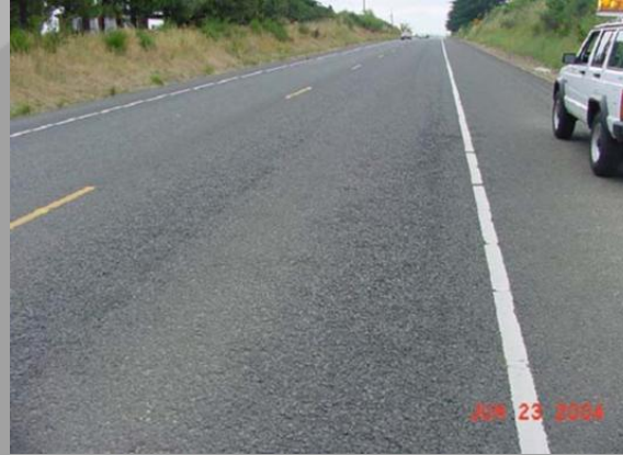
Oxidation and Raveling – Moderate
