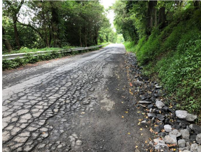
Base Failure
