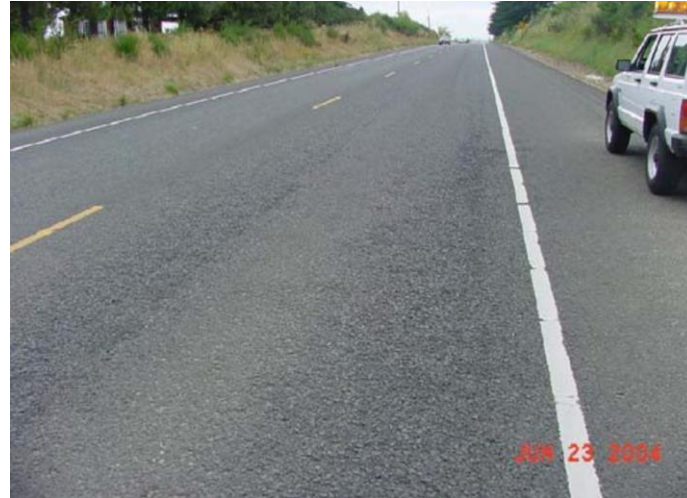
Oxidation and Raveling - Moderate
