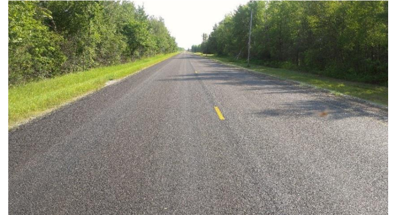
TH 89 after placement of chip seal (2013)
